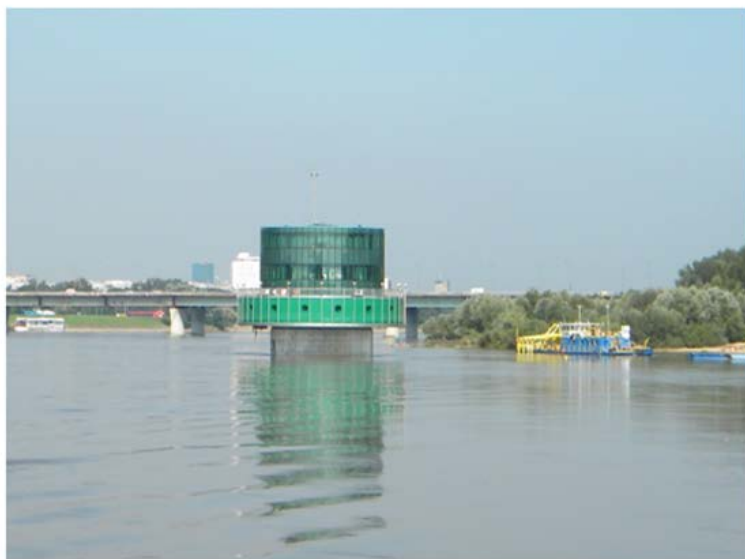
Figure 12. View of "Gruba Kaśka" water intake for Warsaw
